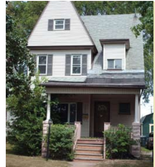
This home on Clinton Avenue was acquired for rehabilitation through the Opportunity Housing program supported by DSCDO.
